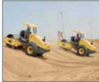
Slope compacting
