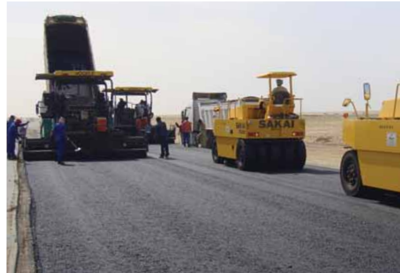
Asphalt laying
