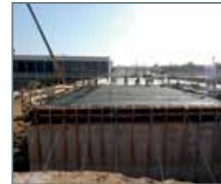
Deck slab form work
