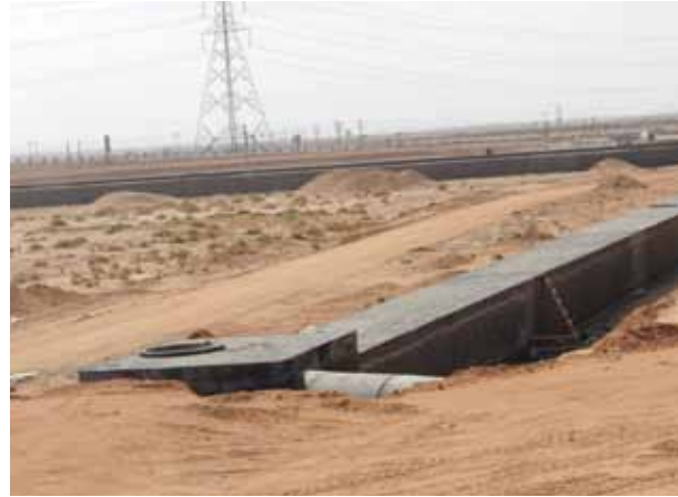
Manhole installation
