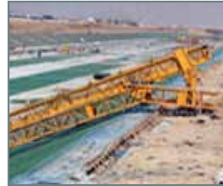
Slope slip-form pavers
